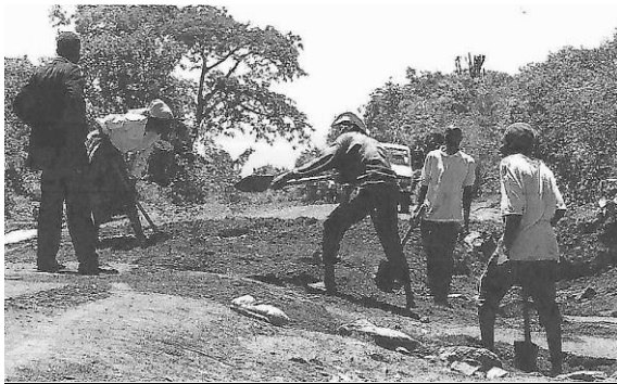
Clearing and leveling
